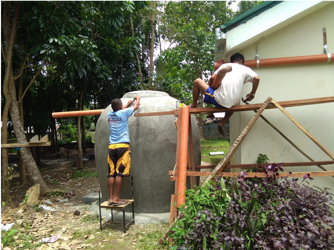
Nearly completed water tank. The extensive roofing of the school-building will fill the tank in 4 hours continuous rain.
