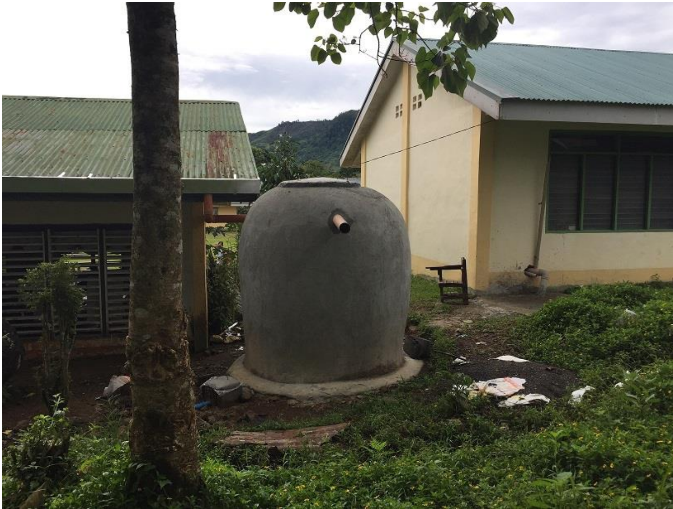
Another rainwater harvester constructed in a school-ground.
